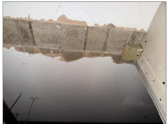
Photo - 19 Shuttered concrete flat roof
