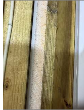
Photo - 25 Insulated plasterboard seen
