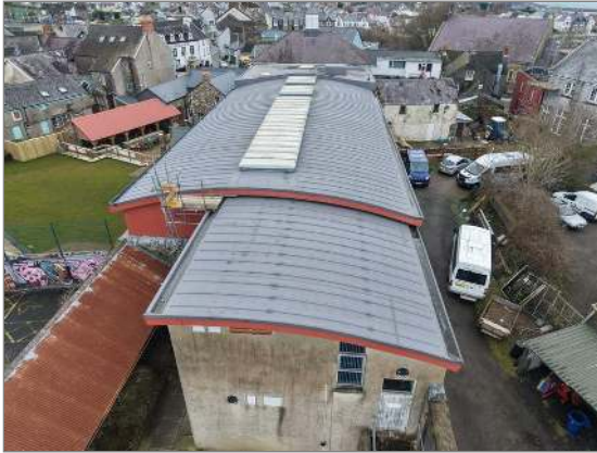
Photo - 2 Aerial view of the building showing the different structures.
