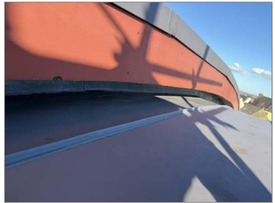
Photo - 11 Flashing/abutment detail for extension roof.
