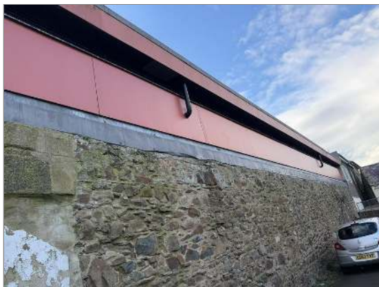
Photo - 13 Lead detail to join where market hall building extended upwards.
