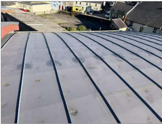
Photo - 10 Aluminium guide rails.
