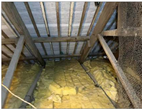
Photo - 16 Roof space
