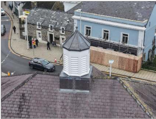
Photo - 4 Original hipped roof and Bell Tower type structure
