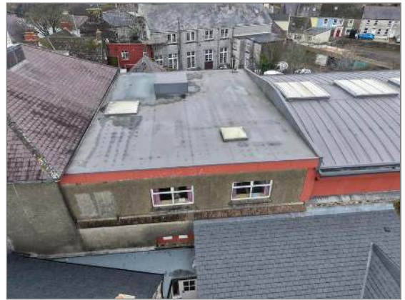
Photo - 5 Flat roof to interconnecting structure.
