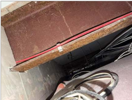
Photo - 20 Steel RSJ for shuttered concrete roof
