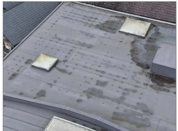
Photo - 7 Circular fixing and ponding.
