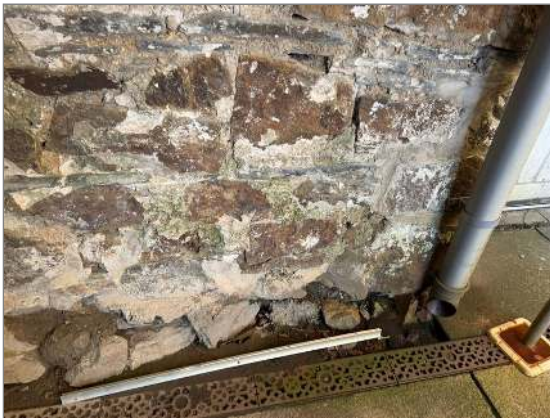
Photo - 15 Repointing works to stone wall to rear of market hall, especially at low level.
