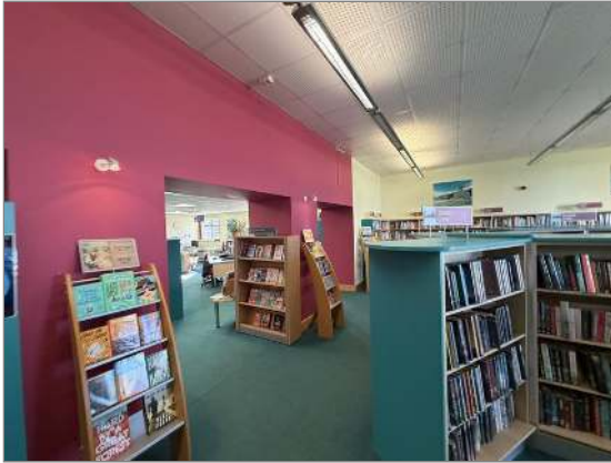
Photo - 24 Parts of the rear original wall has been taken down
